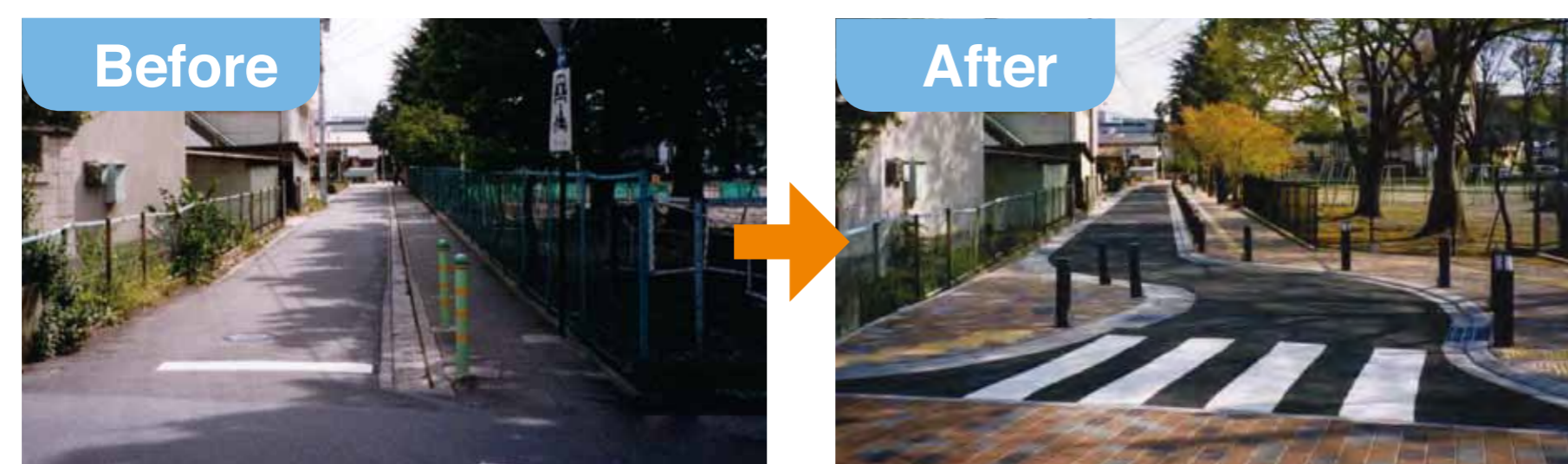
Example of measures to prevent speeding when proceeding to a major road.
