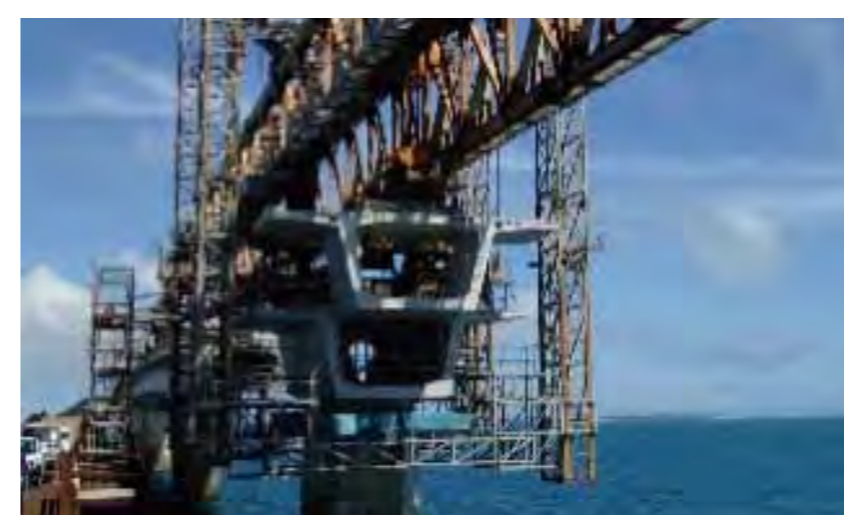
Main girder erection
