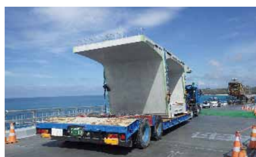
Transportation of main girder along bridge deck
