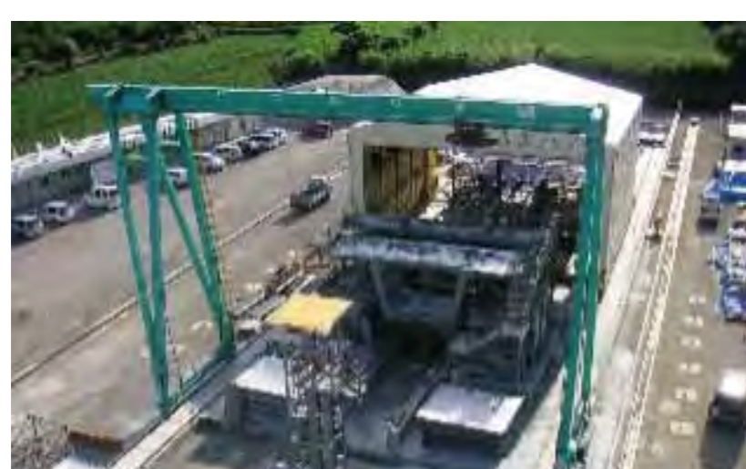
Fabrication of segment at factory
