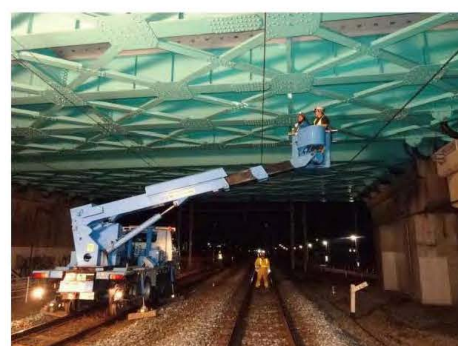
Inspections are systematically carried out for maintaining durability.
