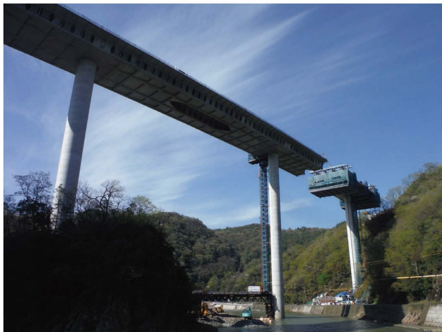
Mukogawa Bridge (Kobe City)
