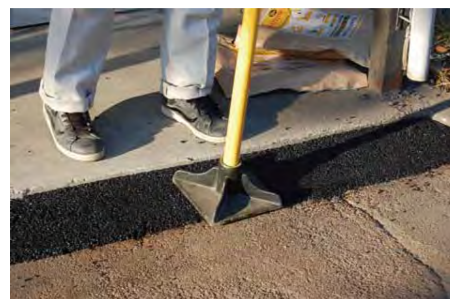
Forming the surface by a trowel, etc.
