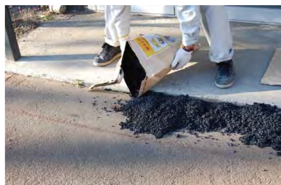
Laying the material after opening the package
