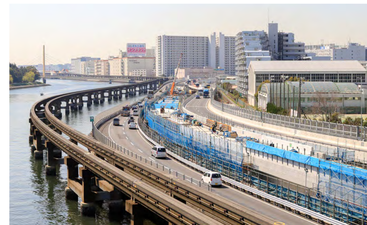
Undergoing Renewal Works (2019)
