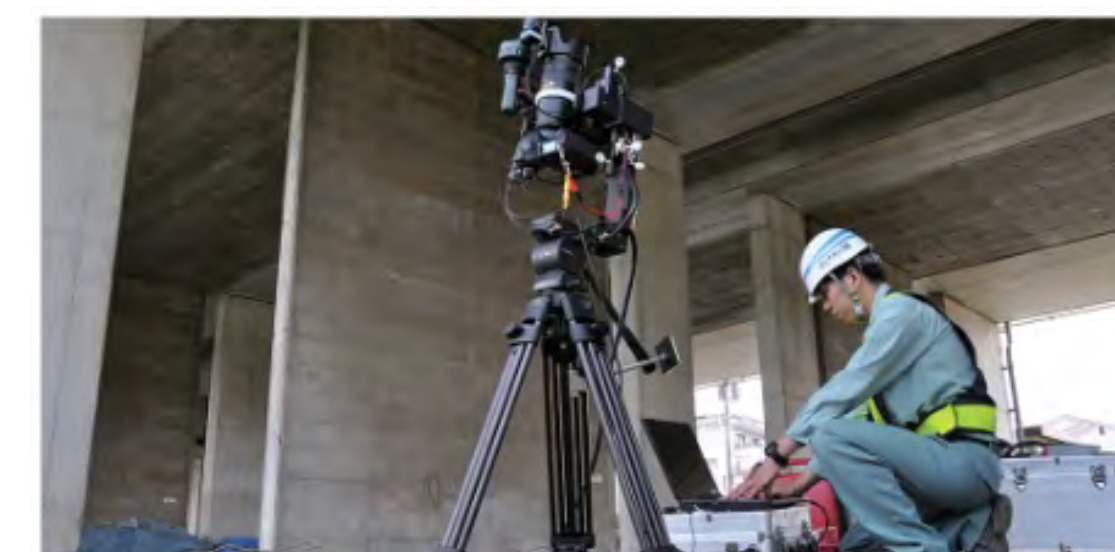
Bridge inspection using Digital Camera System
