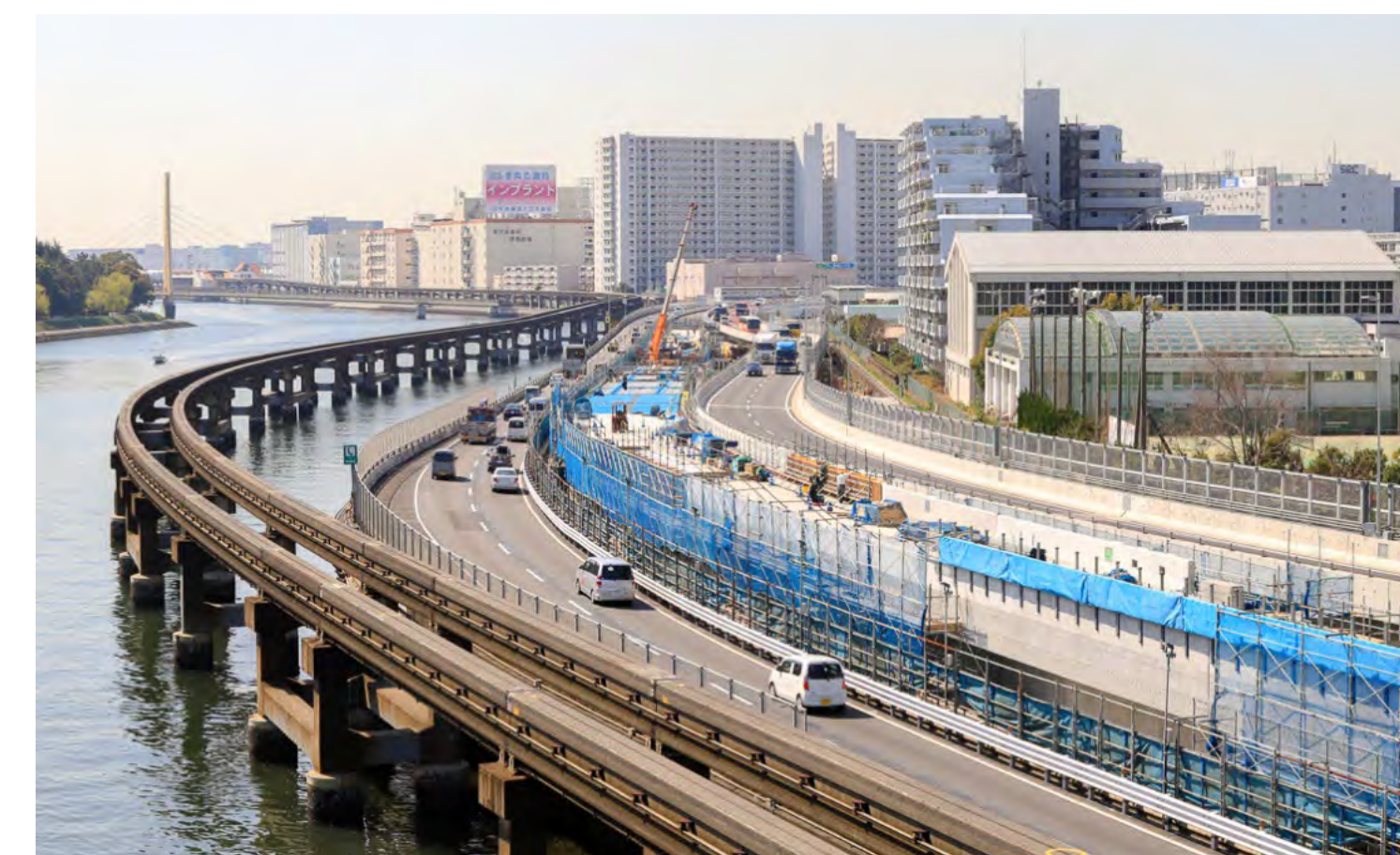
Undergoing Renewal Works (2019)
