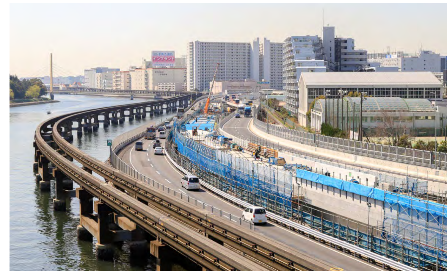
Undergoing Renewal Works (2019)
