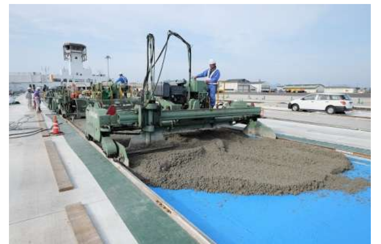
Spreading concrete
