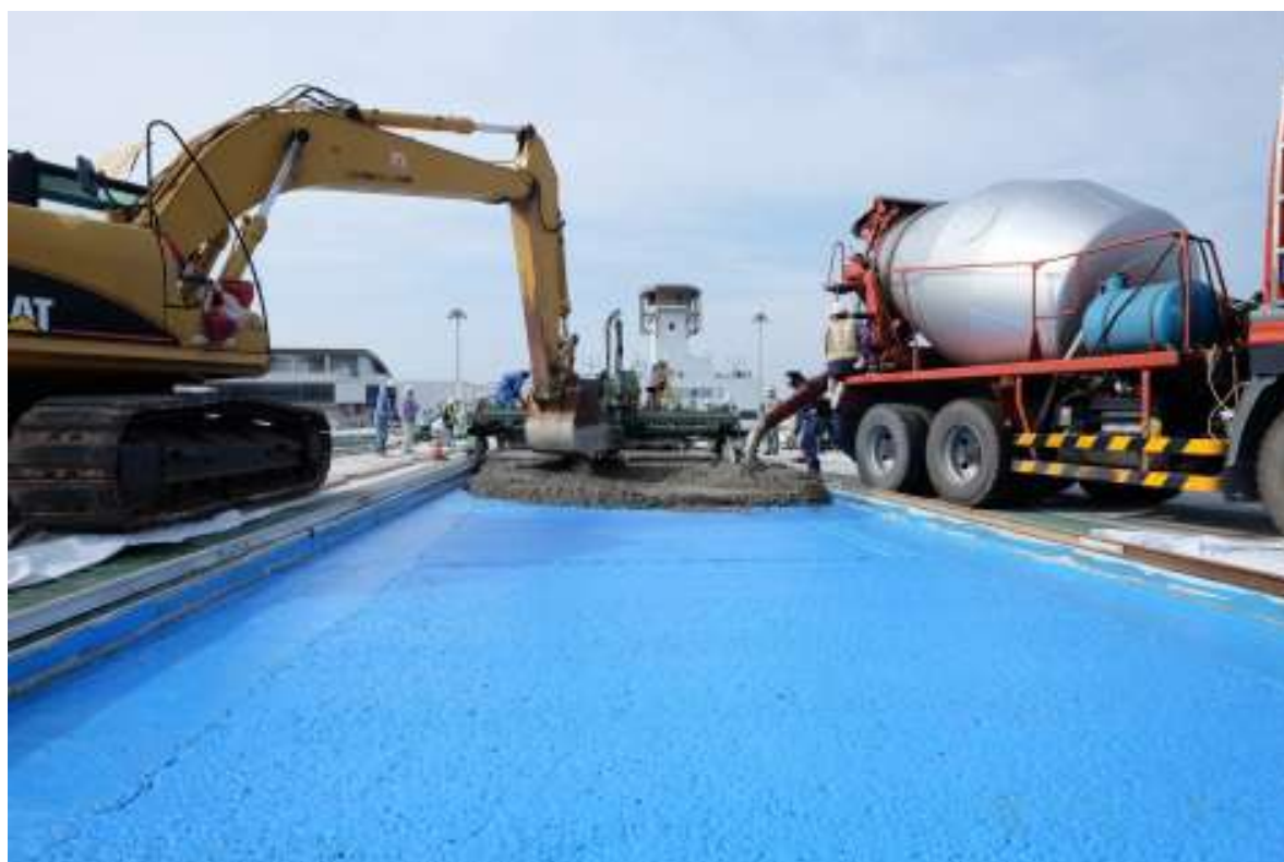
Placing concrete
