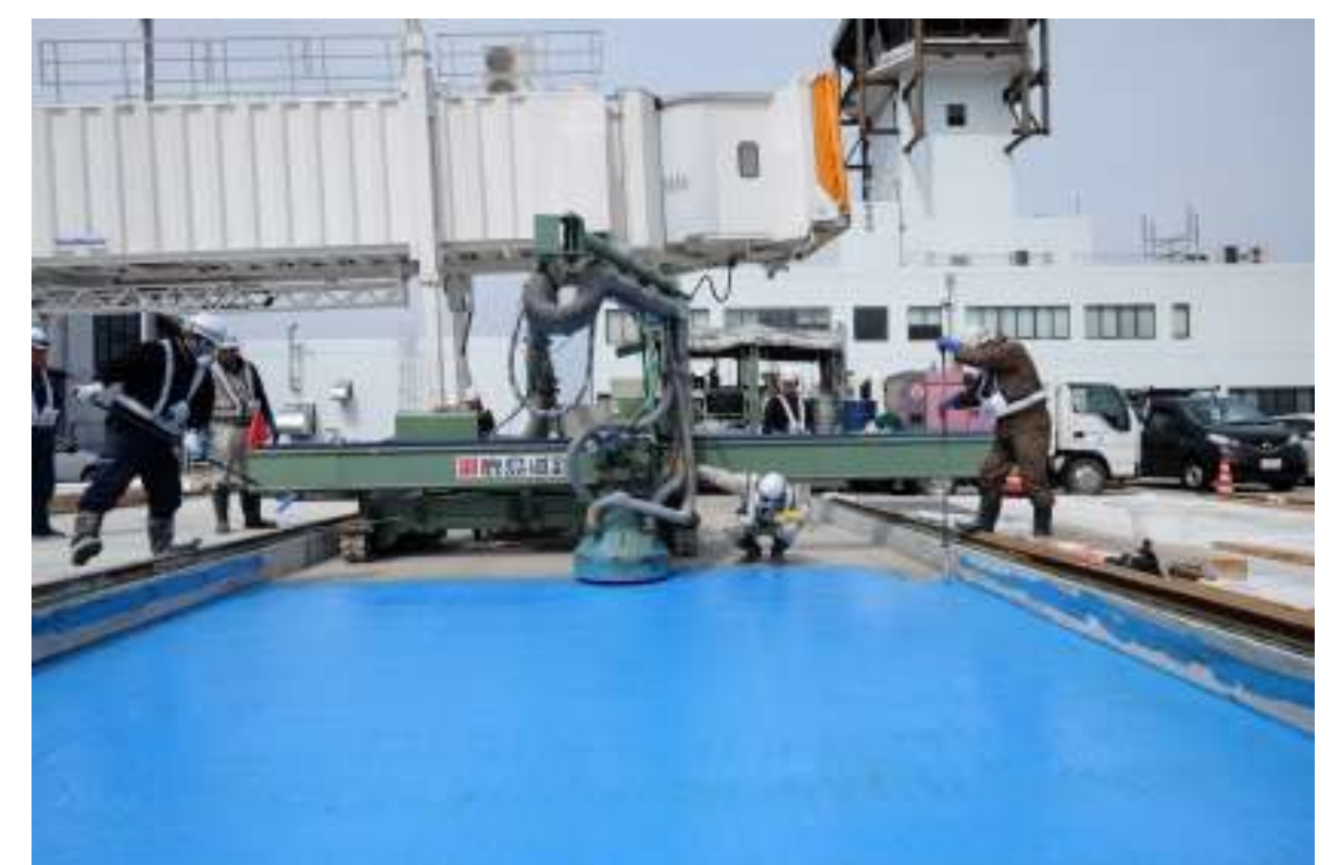
Spraying KS bond-type M
